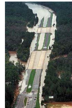
An aerial photograph (left) of State Road 85 looking south shows the extent of the flooding around the Shoal River Bridge, which was closed in 1998.
