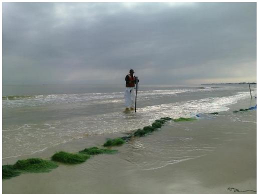
Figure 4.3. Snare booms anchored by posts along the wet beach (USCG, 2010).
