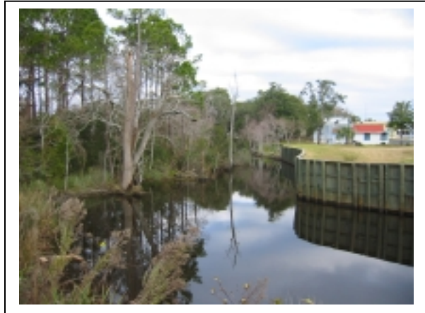
Figure 6-6 Gap Creek Photograph
