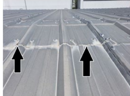
Water Intrusion at the Ridge Cap Metal
