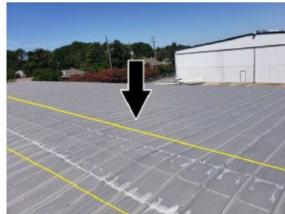
Water Intrusion at the Ridge Cap Metal
