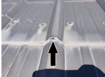
Water Intrusion at the Ridge Cap Metal
